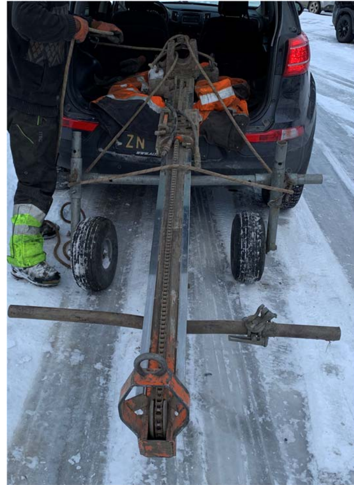
Drilling rig/ setup (Custom made)
